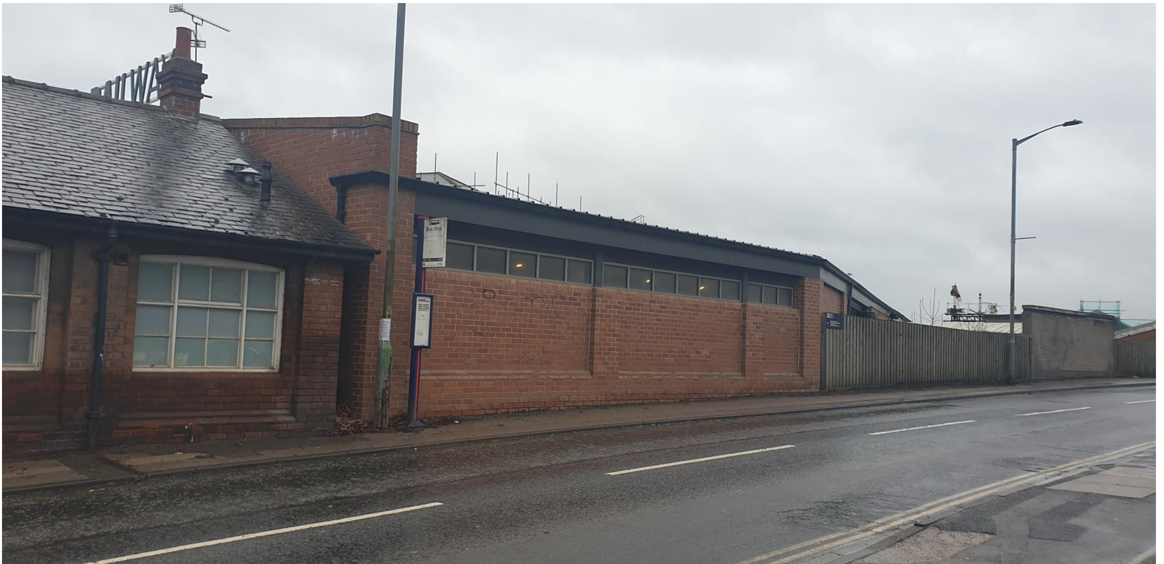
Rear of modern buildings to be demolished
