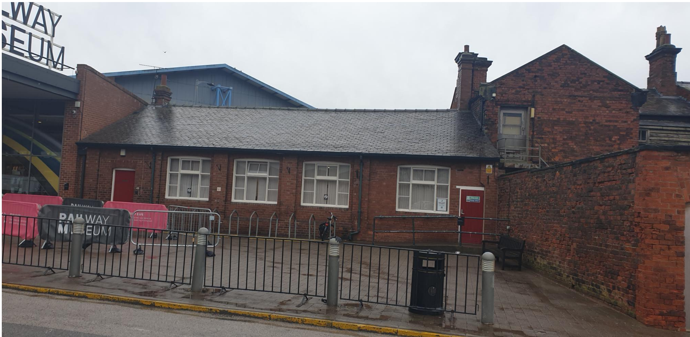
Former mess room to be demolished
