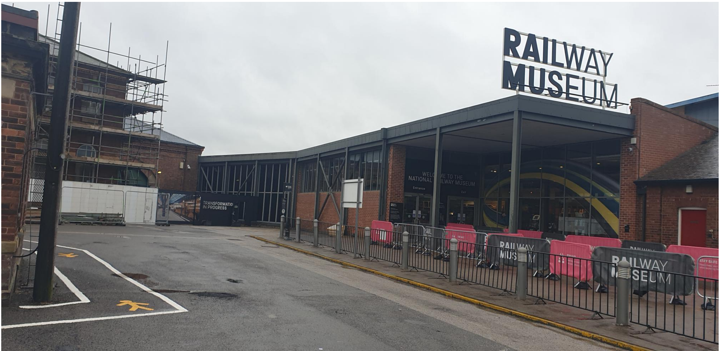
Existing site entrance to be demolished
